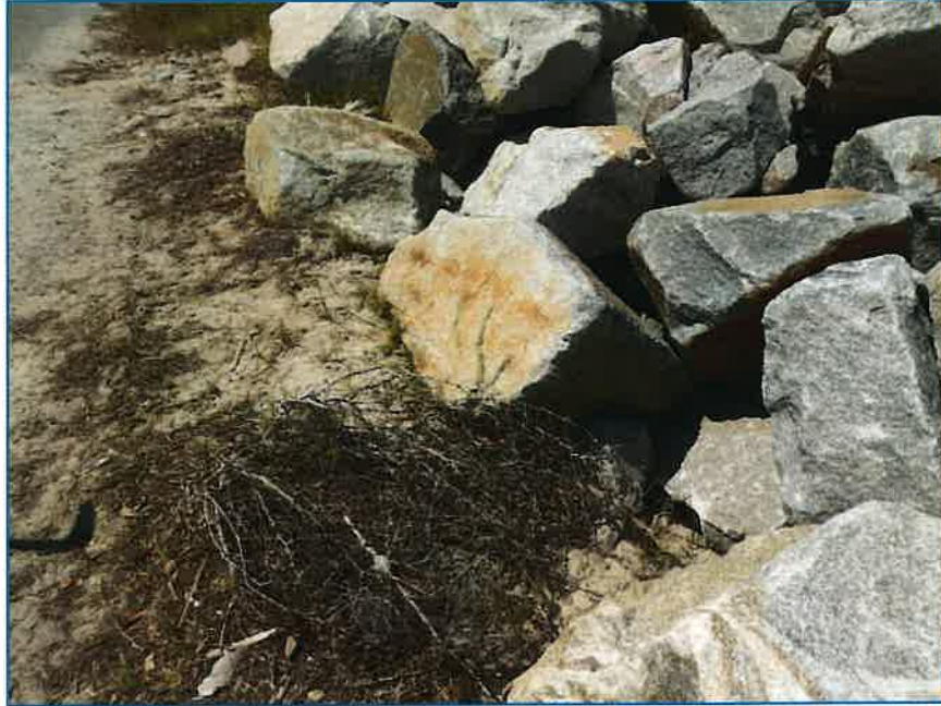
Photograph 5: Station 23+50 – Settlement of Stone Adjacent to Roadway
