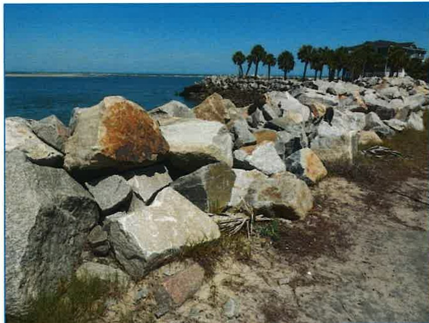
Photograph 4: Station 23+50 to 24+00 - Apparent Settlement of the Revetment
